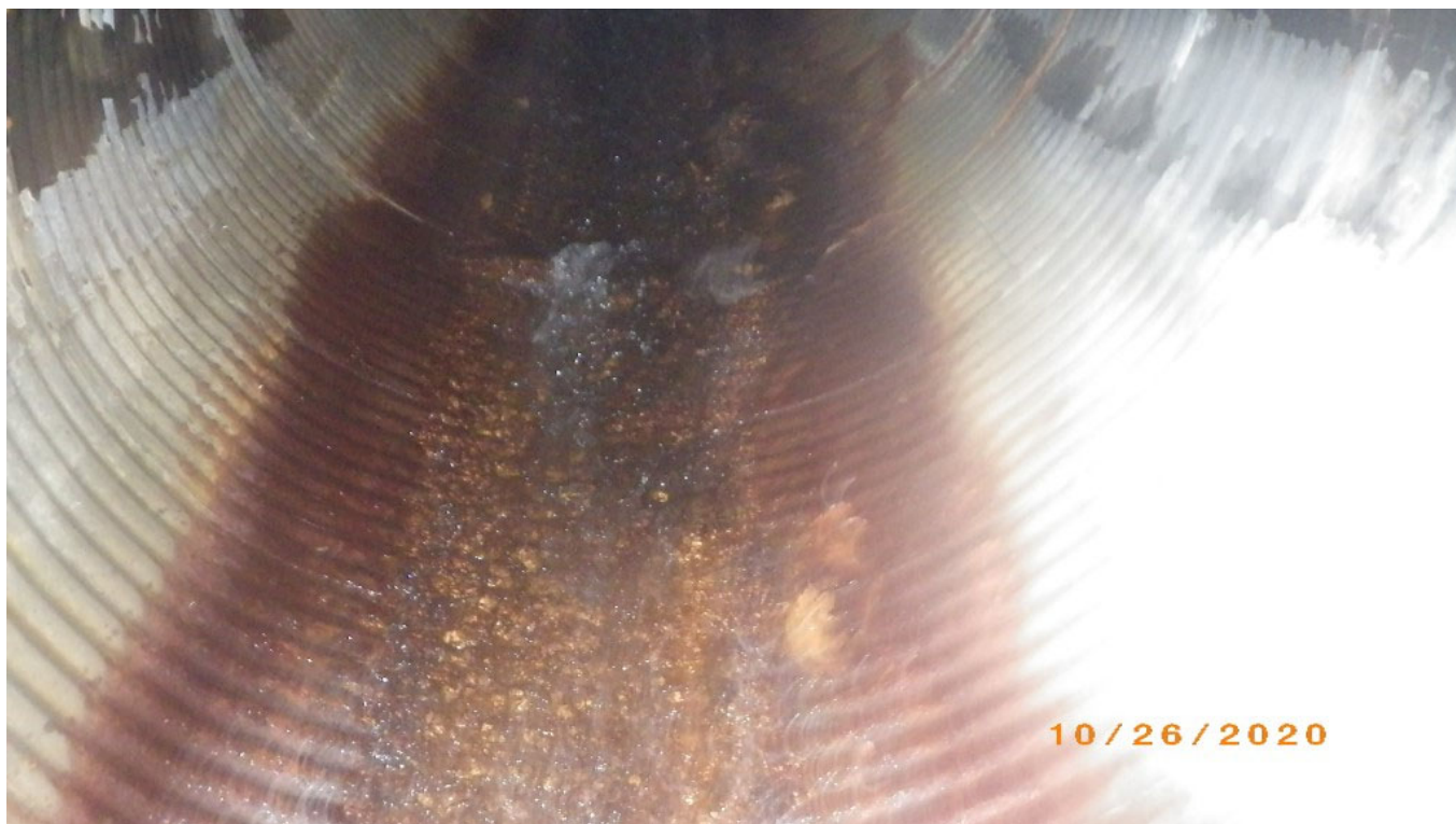
Picture 3: Culvert Barrel
