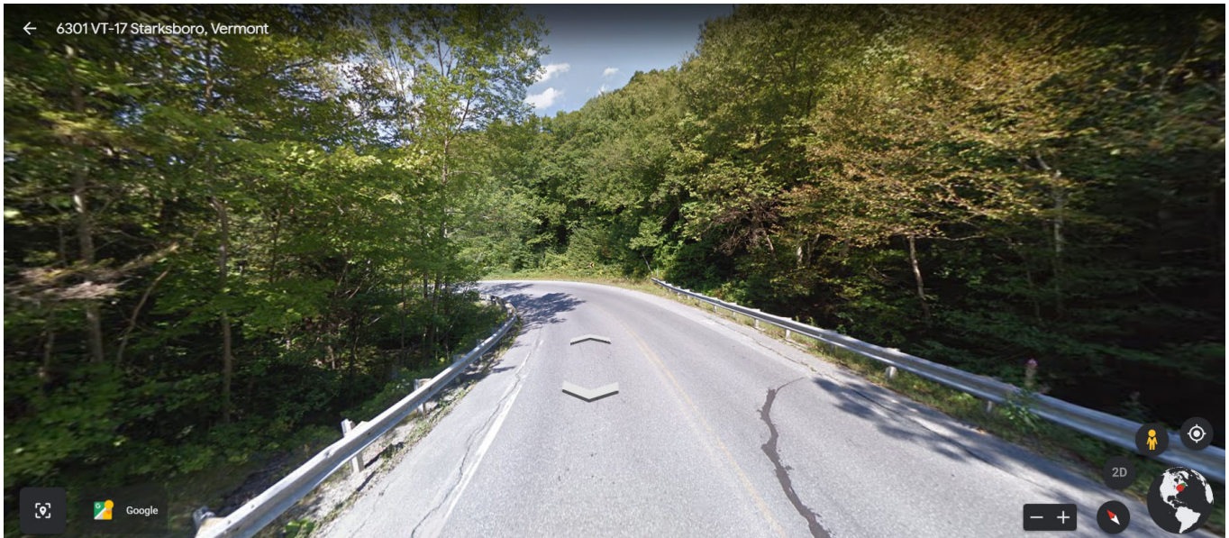
Picture 1: Looking west over Bridge 29
