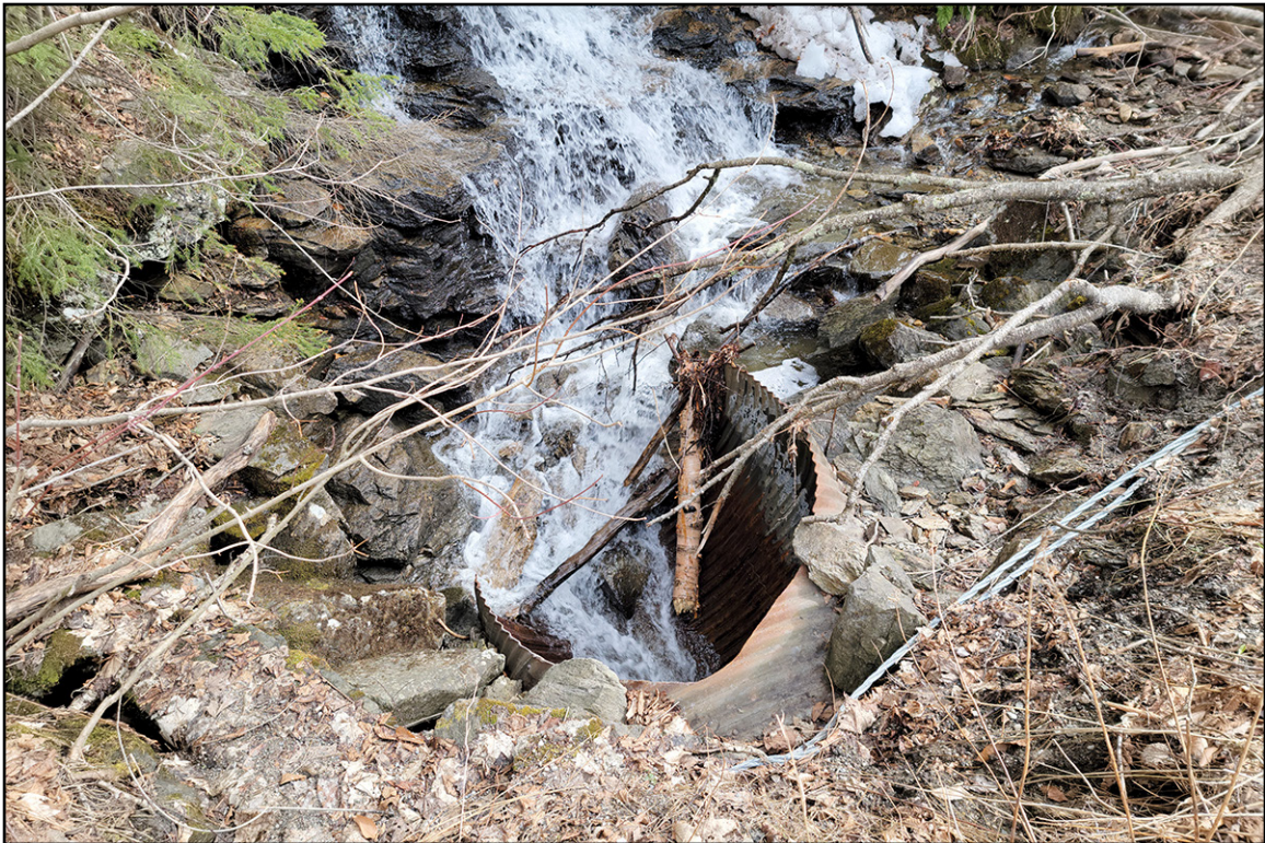
PLATE 2: Buels Gore Culvert No. 29, View of East Side
