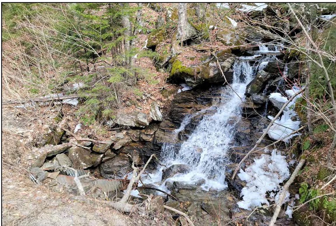
PLATE 2: View of East Side of Culvert, View West
