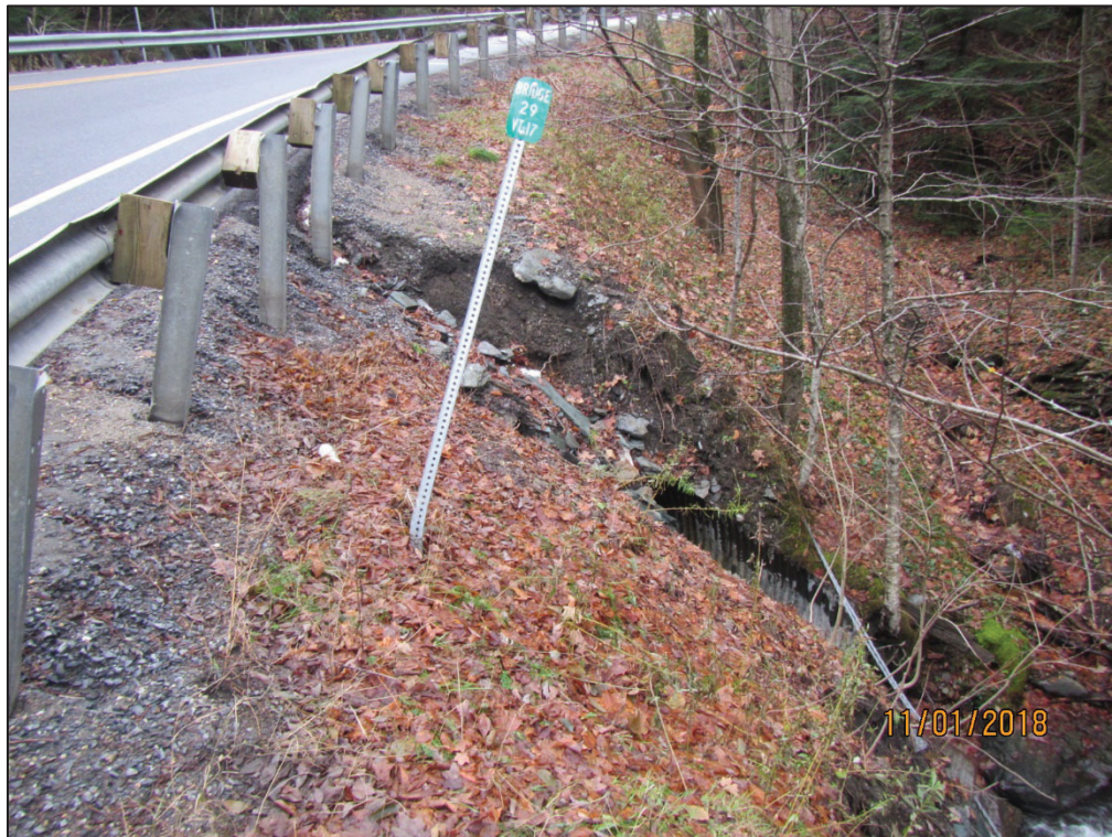
Figure 3.3 Bridge marker and view of the discharging end of culvert. Note the relatively steep grade of the embankments leading down to the culvert.
