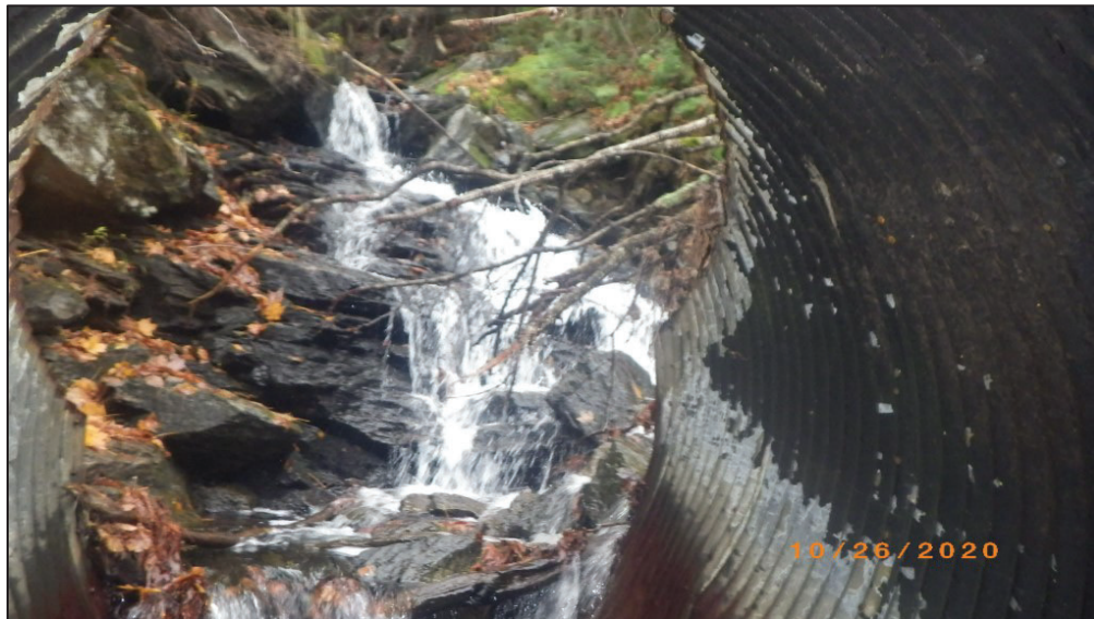
Figure 3.1 Looking upstream from within the culvert at the stream. Note presence of bedrock outcrops and loose blocks.
