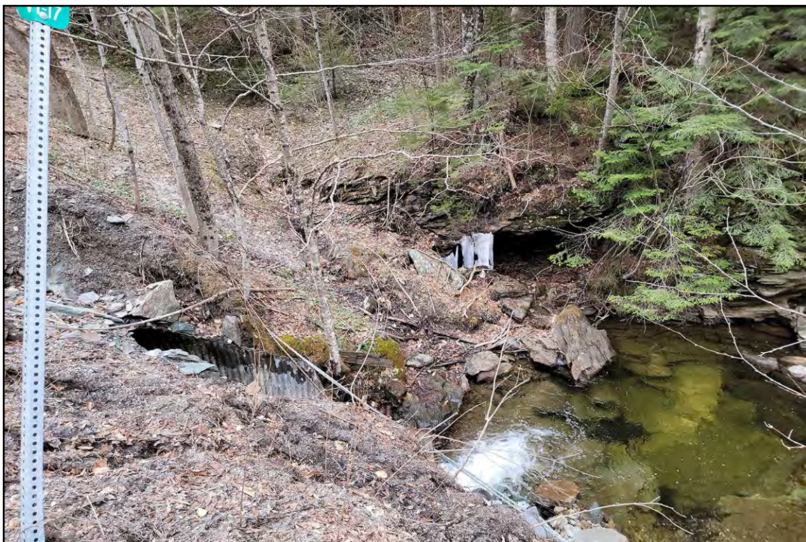
PLATE 1: View of West Side of Culvert, View East
