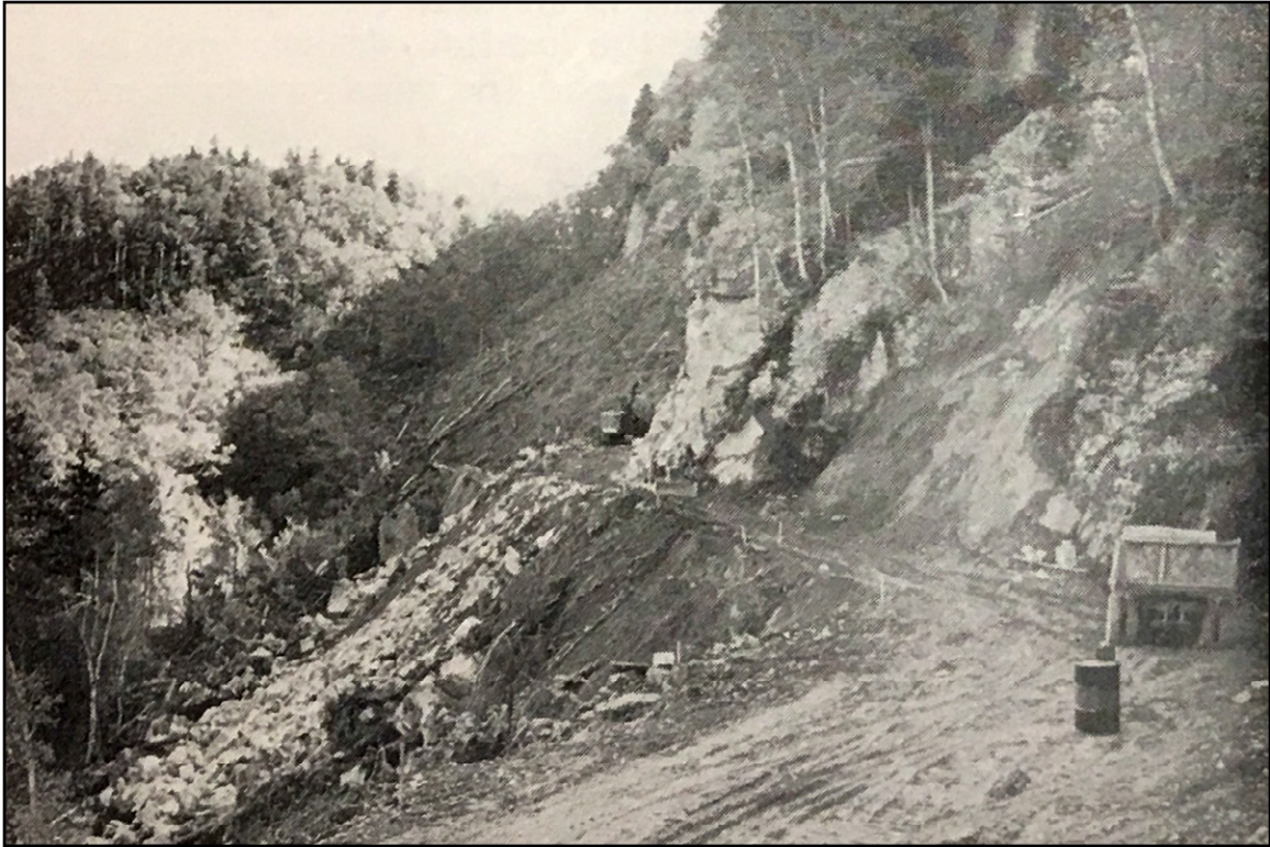
FIGURE 4: Excavation for McCullough Turnpike Connector (Vermont State Highway Board 1954-1956)
