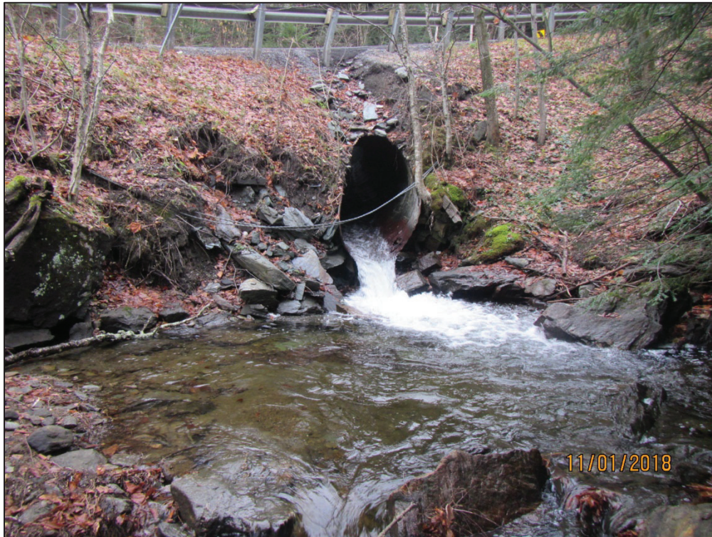
Figure 3.4 Discharging end of culvert. Note probable bedrock around base of culvert.
