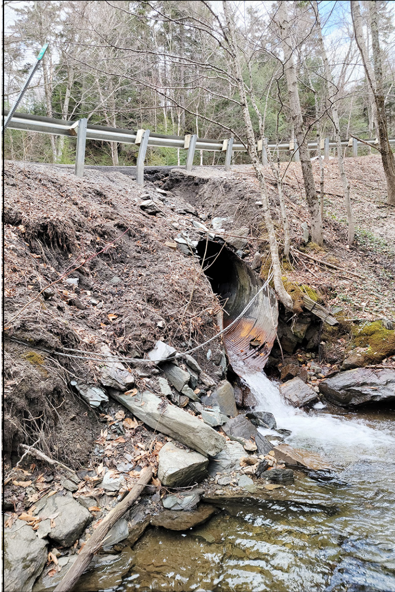
PLATE1: Buels Gore Culvert No. 29, Facing Southeast
